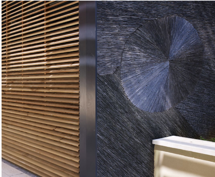
12 Cladding details at the building entrance, including louvers at different scales. Varying rotations of the louvers cast shadows, giving a layered effect to the facade.
