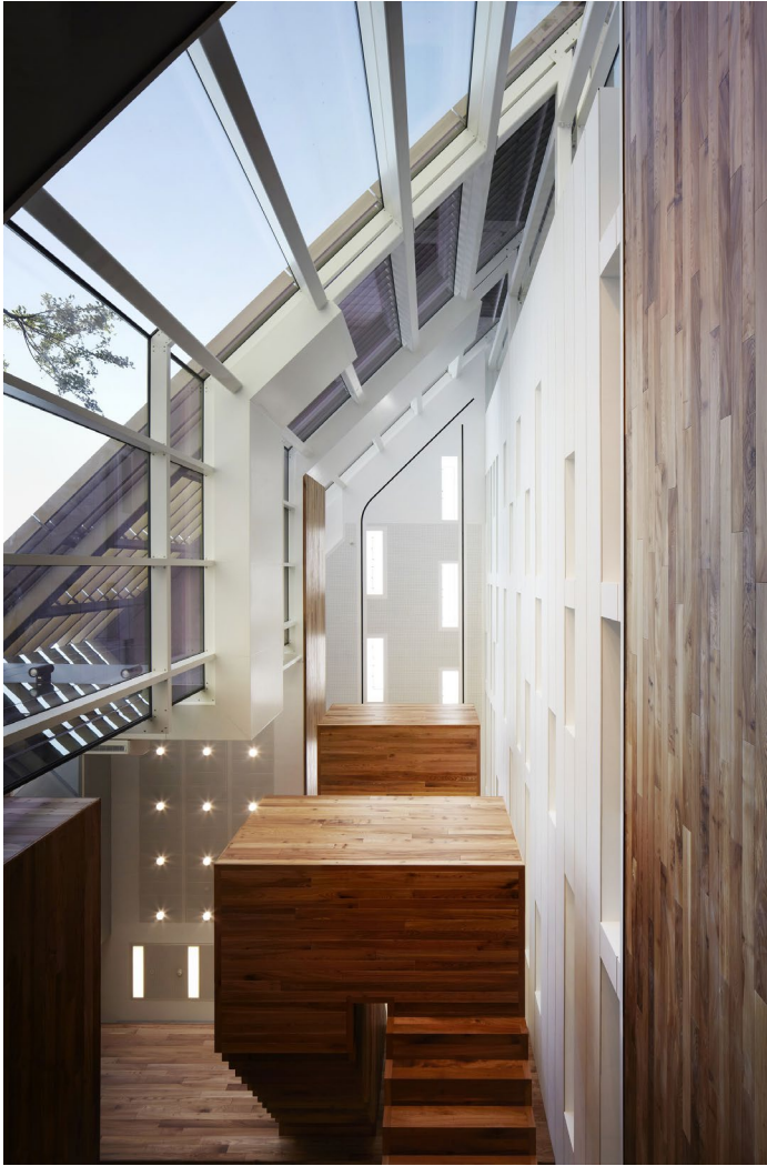
9 View looking up to the top of the atrium. A prominent sawtooth configuration on the underside of the staircase follows the lines of treads and risers above.
