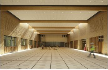
18 Dining hall nearing completion. Brickwork 'screens' on either side of the hall provide openings for return air and acoustics.
