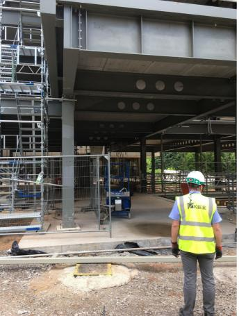
18 Steel frame of the Learning Hub under construction. All the major building components were prefabricated, including the steel frame, the cross-laminated timber, and the concrete and rainscreen cladding.
