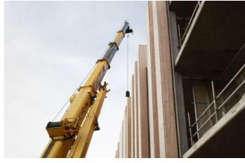
6 Construction images showing the straw panels being installed on site. Each panel spans all four floors of the building in one prefabricated piece.
