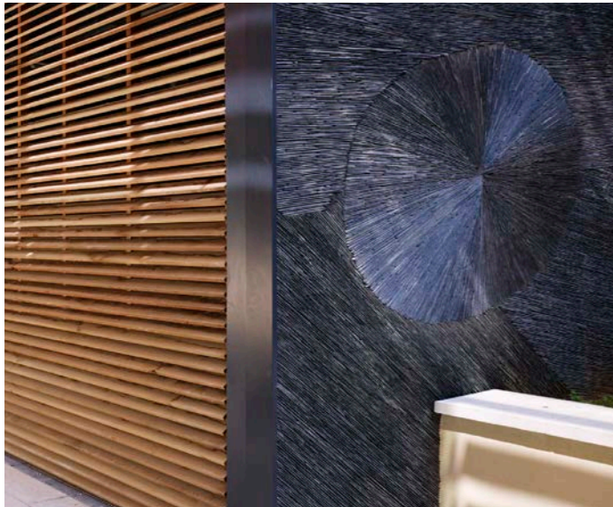
12 Cladding details at the building entrance, including louvres at different scales. Varying rotations of the louvres cast shadows, giving a layered effect to the facade.
