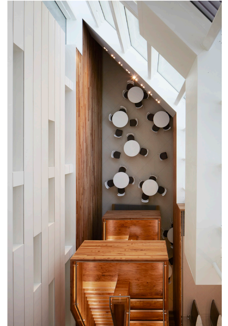
10 View down through the atrium. A stainless steel handrail wraps around the internal faces of the stair to provide a visual contrast with the warm texture of the elm.
