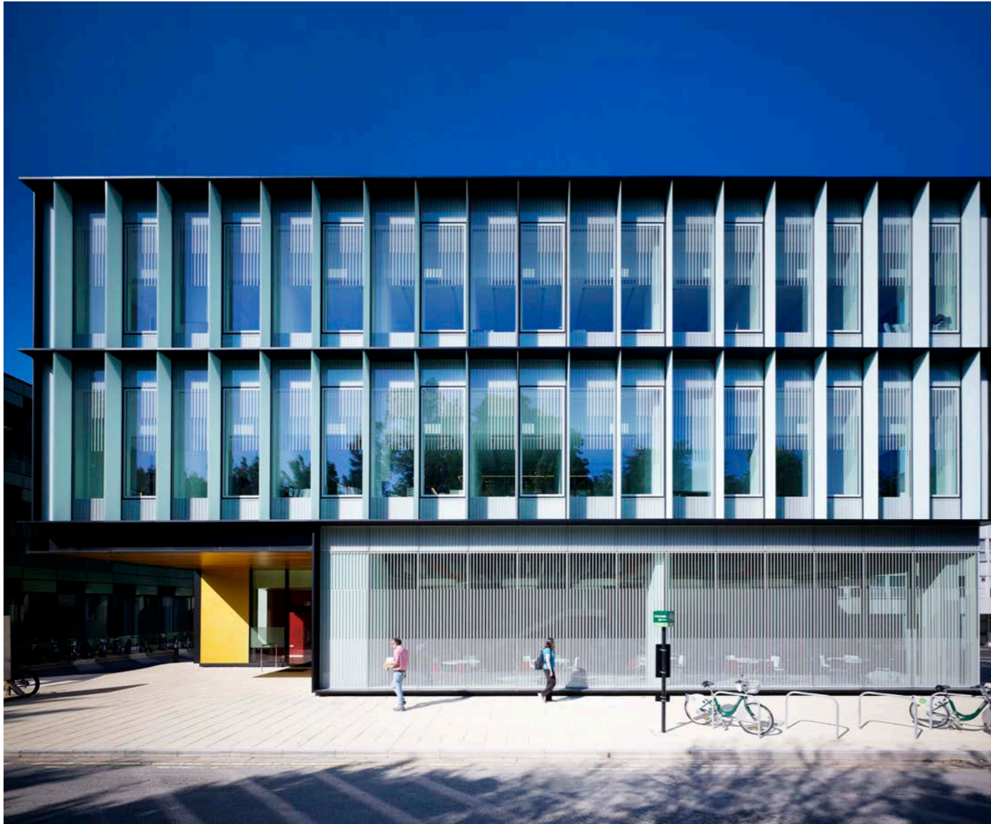
11 East elevation showing the café space at the lower level, with offices above that feature outward-opening windows.
