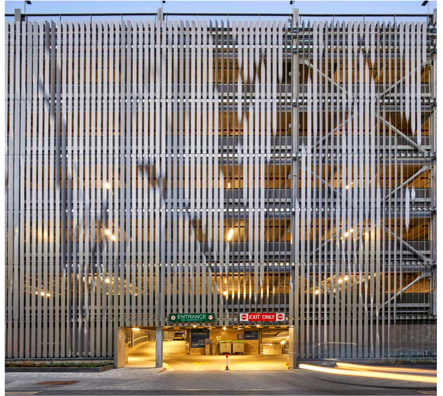
12 Main entrance/exit to the multi-storey car park. A digital script was used to define specific twists in the aluminium blades to give the appearance of tree silhouettes across the facade.
