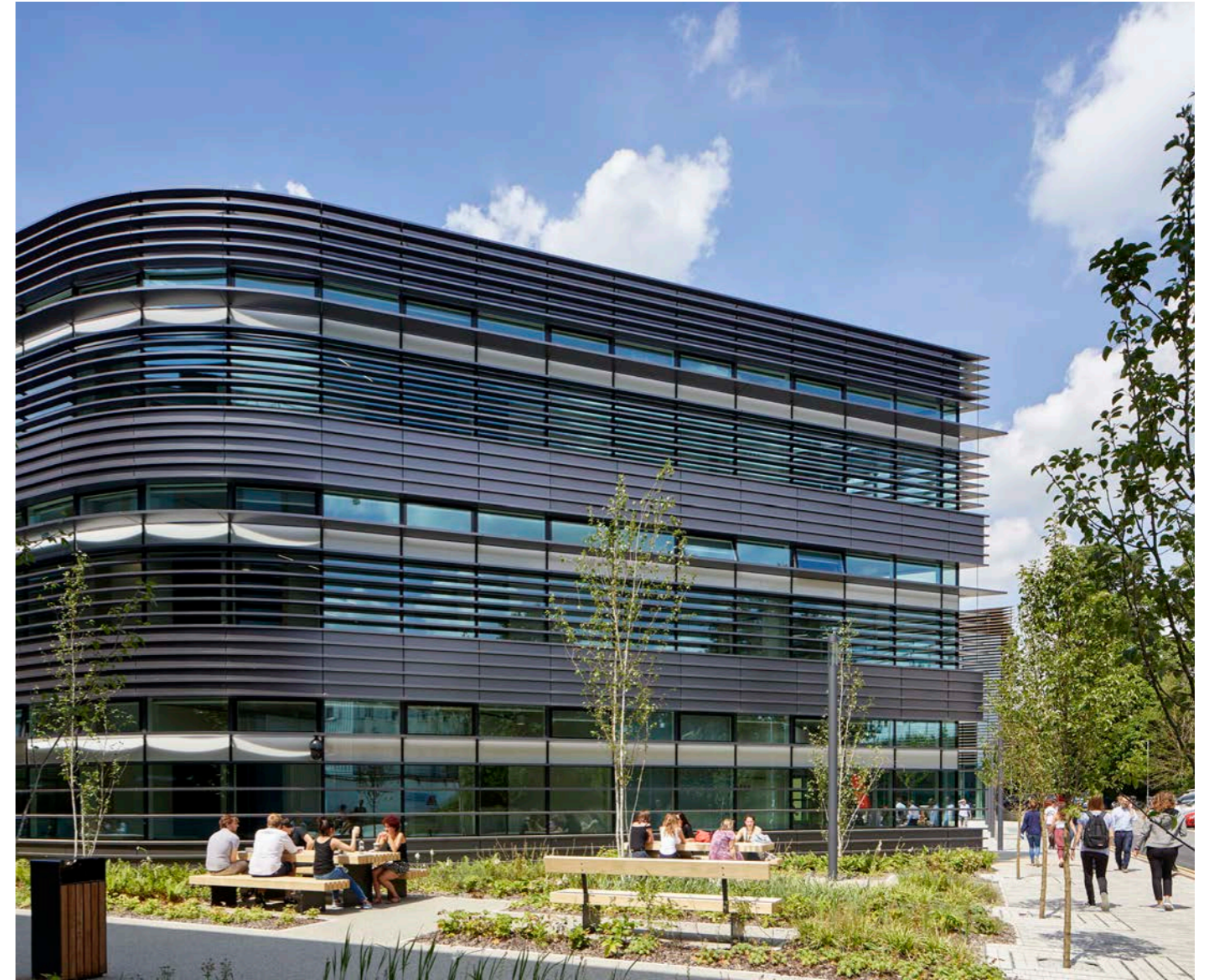
8 South-east approach, where the articulation of the building form has enabled the inclusion of several informal planting areas.
