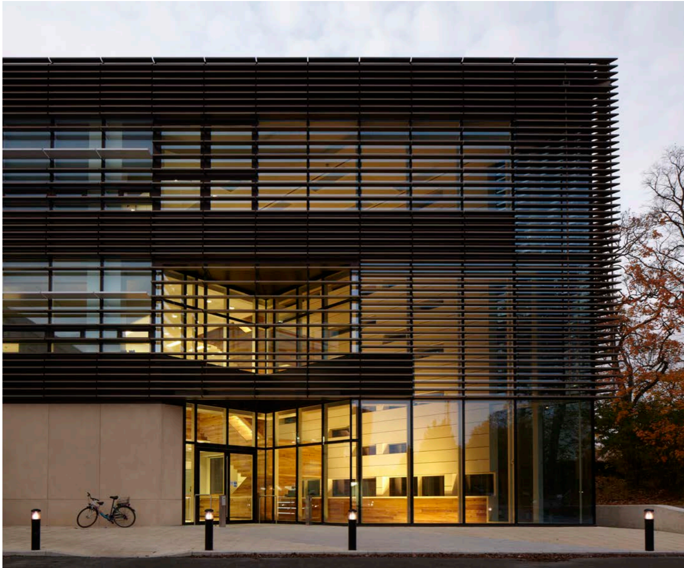
7 South elevation showing the horizontal louvers cladding the building. The slot windows and rooflights project varying patterns of natural light into the building's interior, creating energising contrasts of sunlight, shadow and shade.
