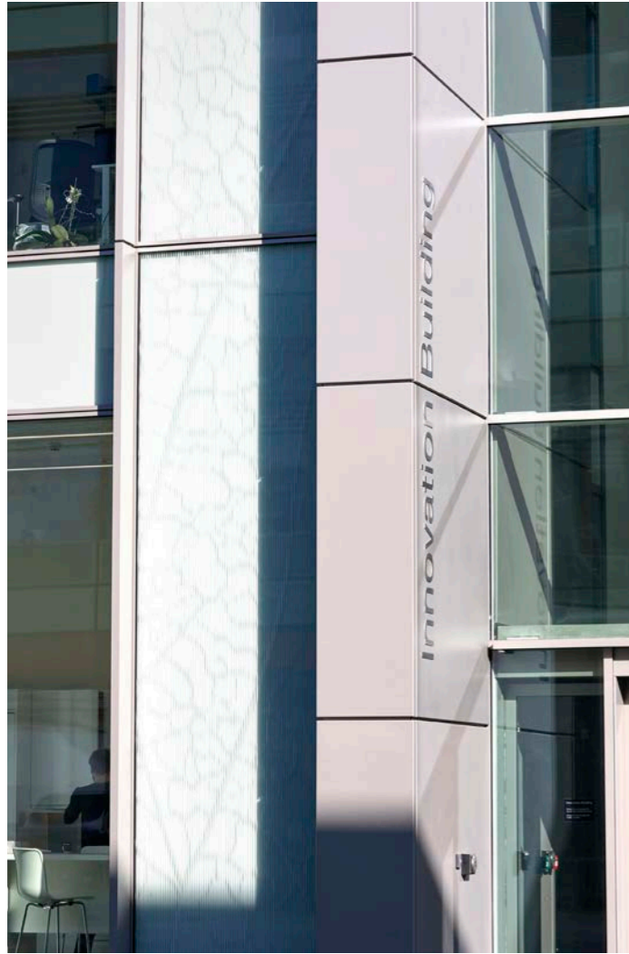
13 Main entrance with projecting fin that separates the building's different functions.
