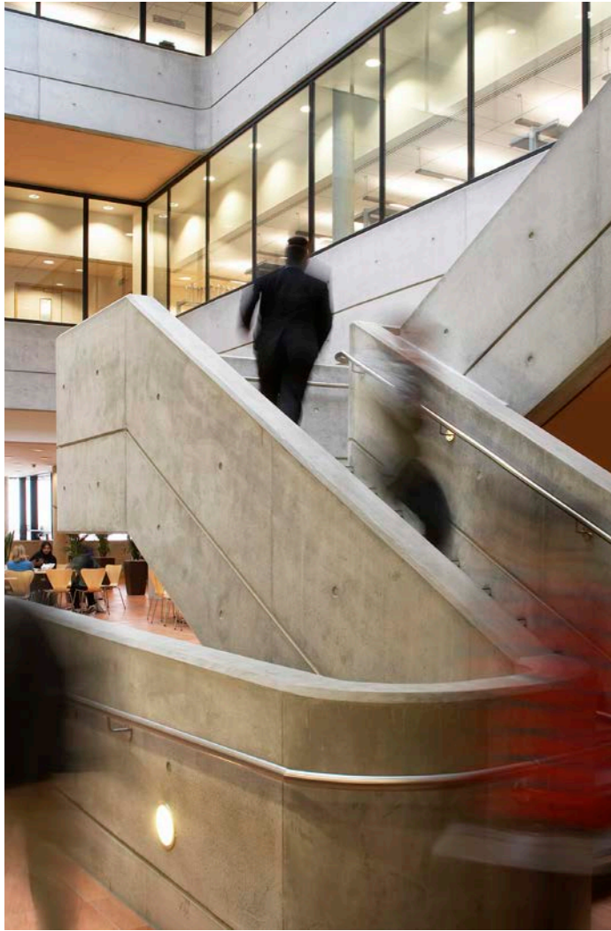
12 Atrium staircase with cast in-situ concrete. The building's social heart includes a café and a knowledge centre.
