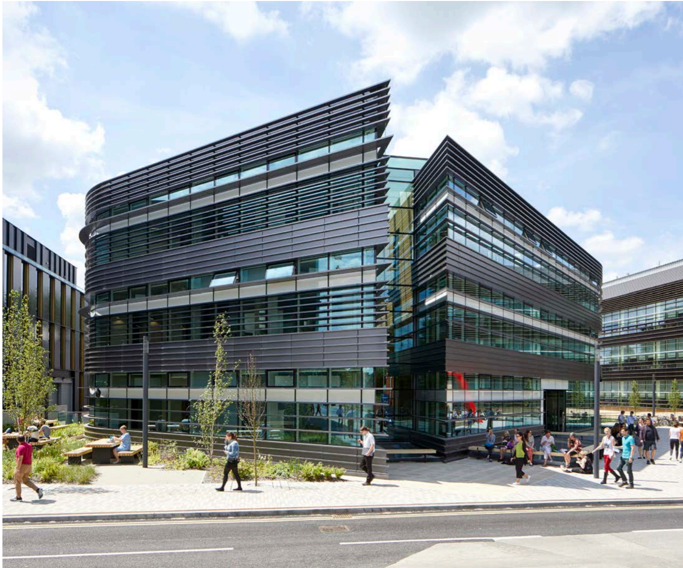
7 Approach from the main road, with formal landscaping. The facade draws on the horizontal cladding of the neighbouring NDM Research Building, with a veil of grey polyester powder-coated aluminium bands and glazing.
