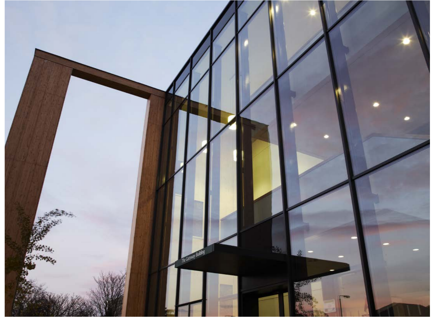
13 Entrance atrium and gateway upon completion.
