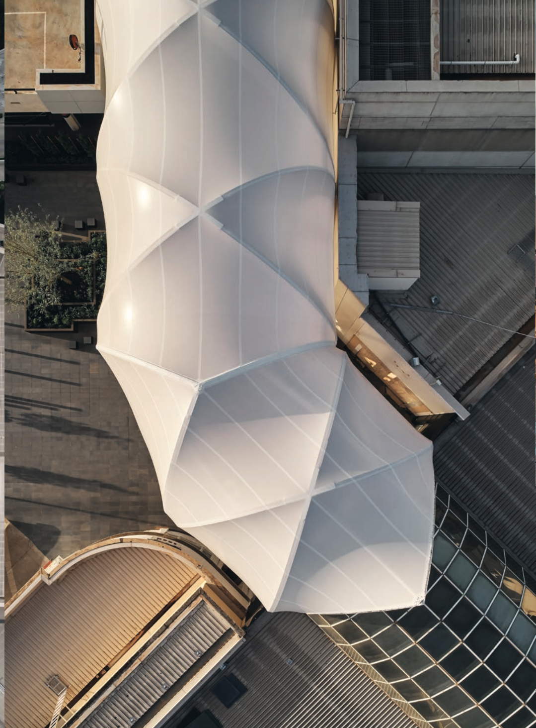
4. The vaulted diagrid structure of the Link, which references the dramatic arched glass roof of the shopping centre.
