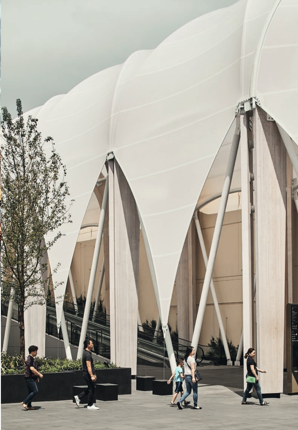
6. Entrance during the day, with view of the stairs, travelators and soft planting. The open sides allow for cross-ventilation, eliminating the need for air conditioning.
