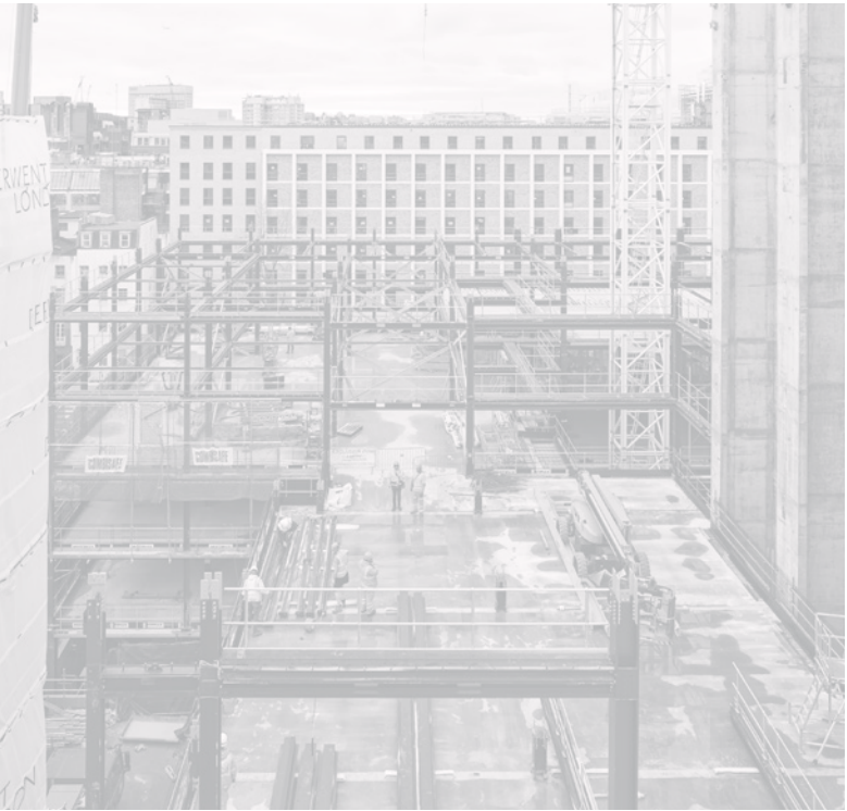
2. An expressed steel frame is arranged around the development's central jump-form core.
