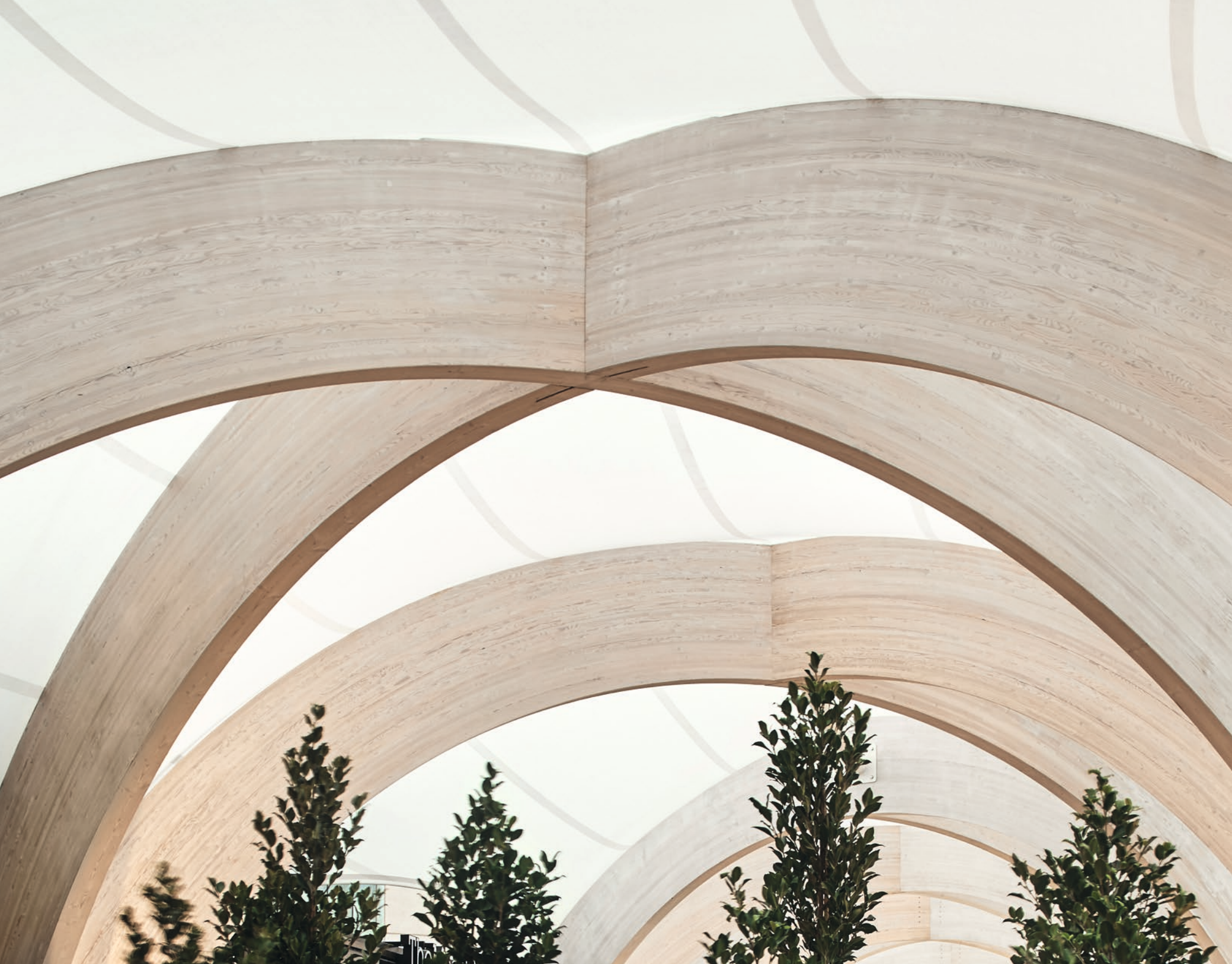
10. Detailed view of the structure, which contains 100 pieces of glulam that create 30 arches, connected with concealed metal plates. Three pieces of PTFE fabric, each 40m long, were stretched over the structure after each section was built.
