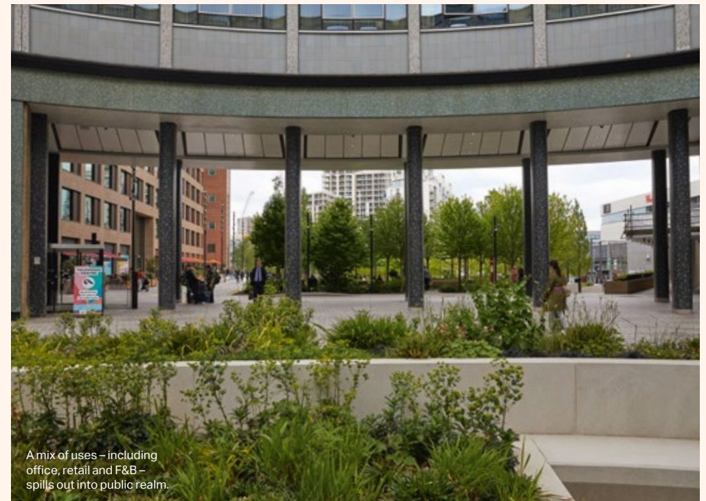
The former BBC television studios are the centrepiece of the White City development.
