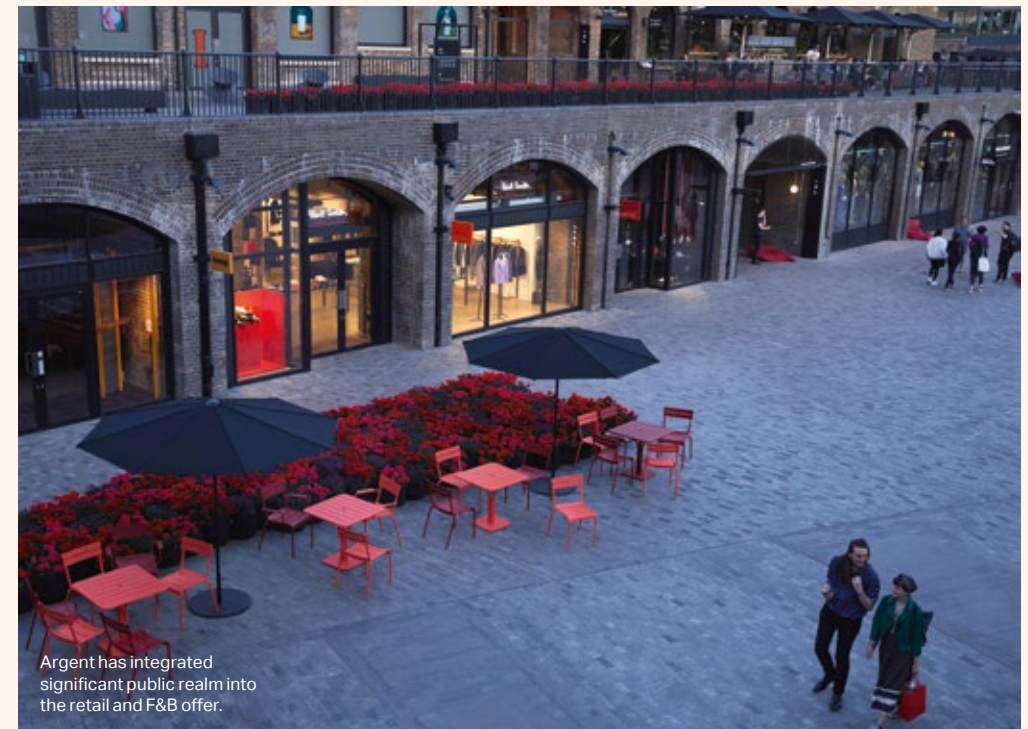
Victorian brick viaducts and industrial sheds have been reimagined and extended in a social-media savvy design.
