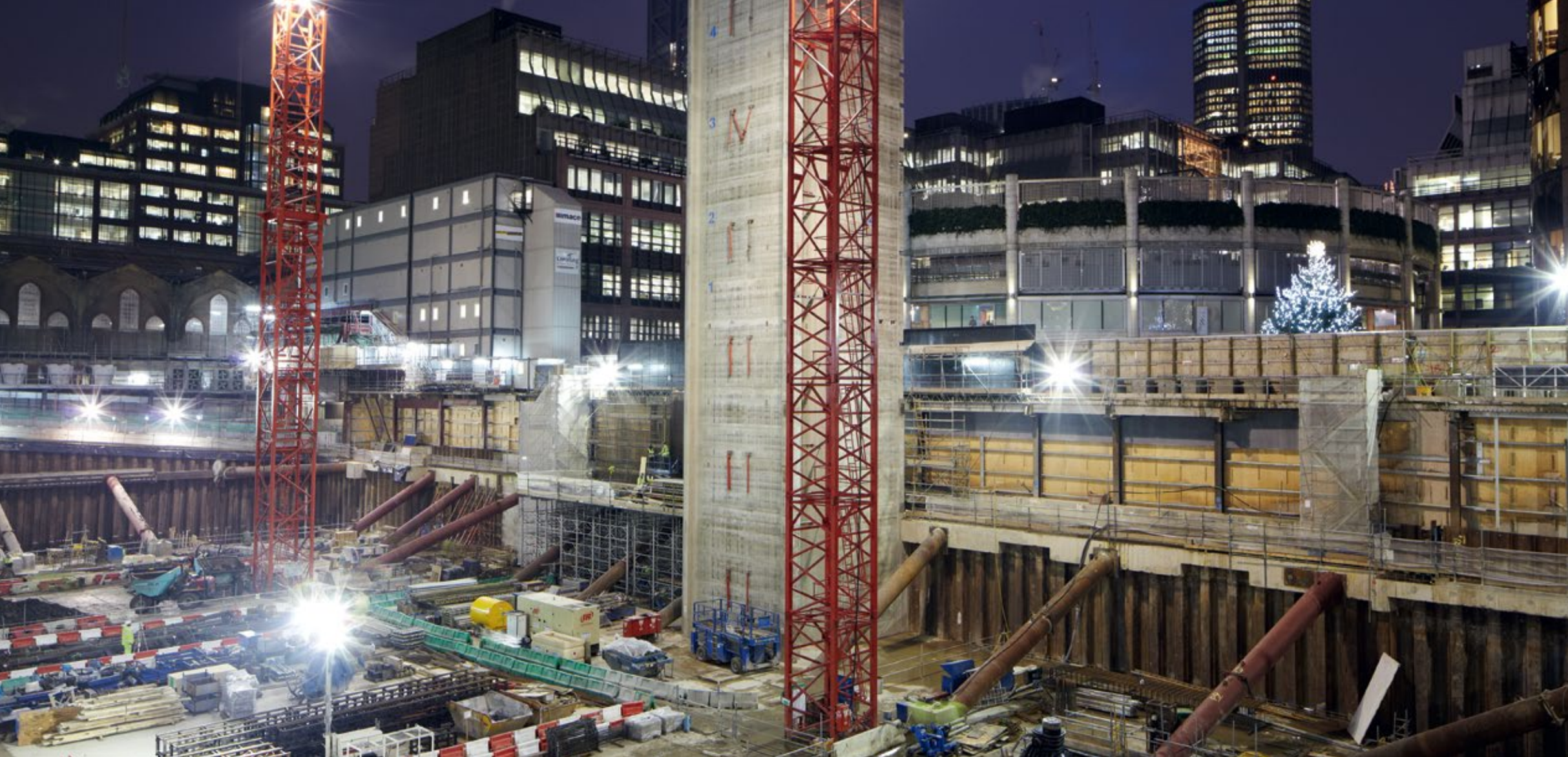
1 Night-time photograph of the ground and core works.
