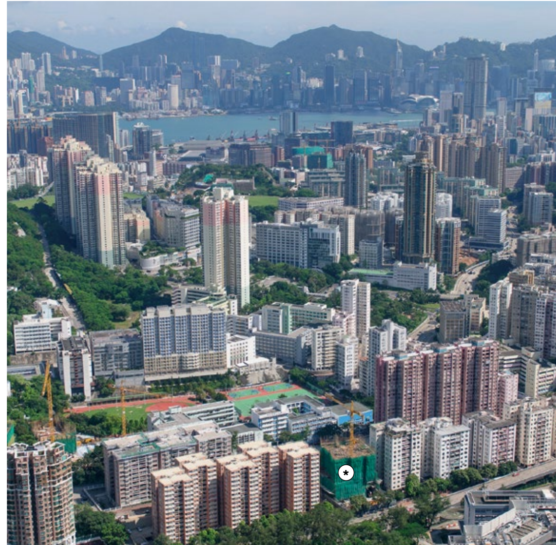
1 Aerial view of Kowloon showing the Argyle Street tower under construction.
