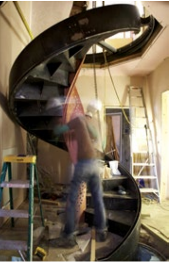
The stunning spiral staircase, made from patinated brass, aluminium, toughened glass and oak, was prefabricated in the warehouse, then taken apart and reassembled on site.
