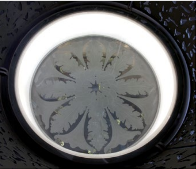
This 'oculus' (right) creates an opening which links two floors; the pattern etched into the sandblasted glass originates from an existing ceiling rose.
