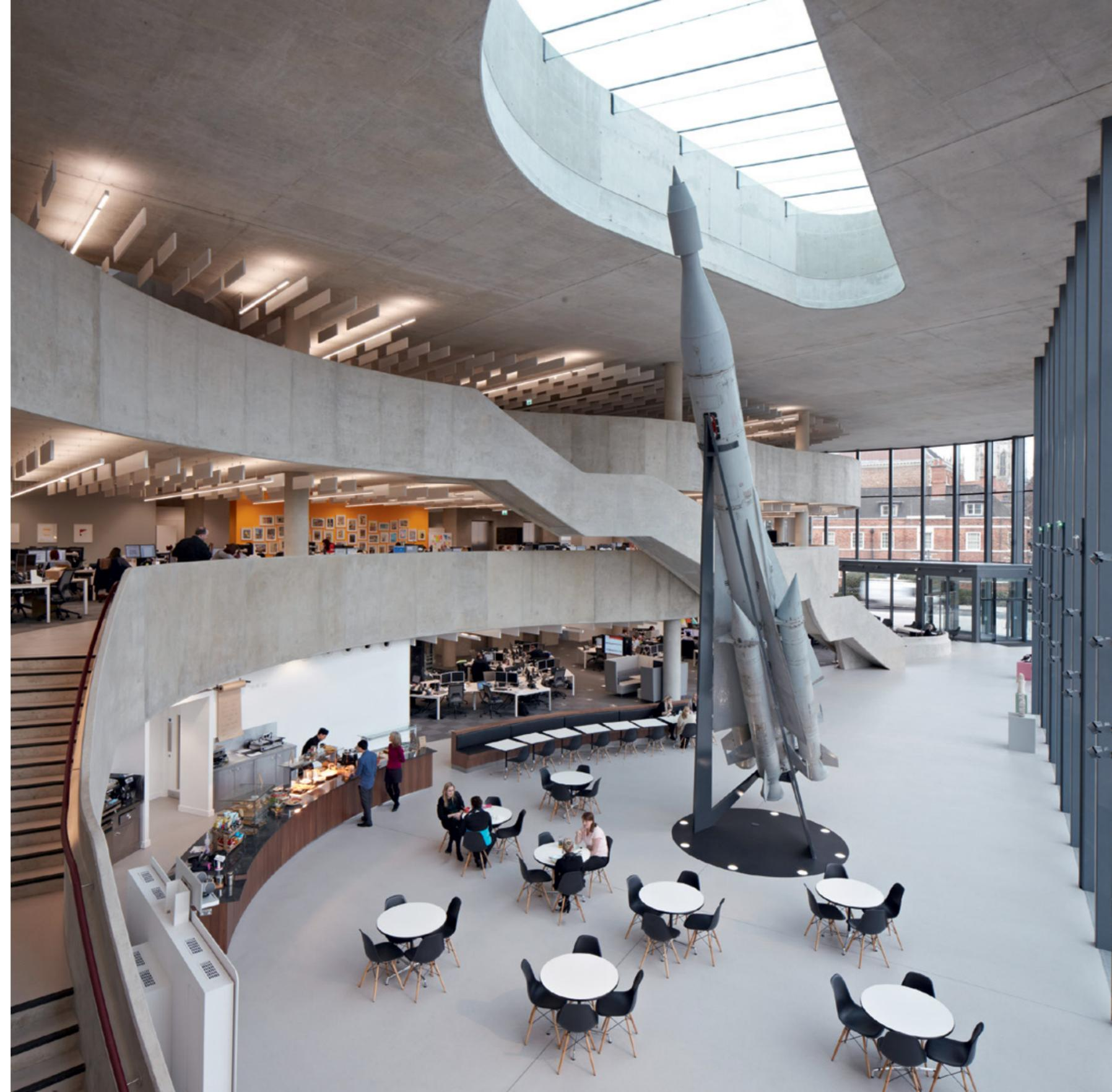
**1 (Previous spread)** The building is made with 5,000m<sup>3</sup> of concrete – enough to fill two Olympic-sized pools – forming the piled foundations, superstructure, feature staircase, balustrades, escape stairs and brick-faced facade panels.
