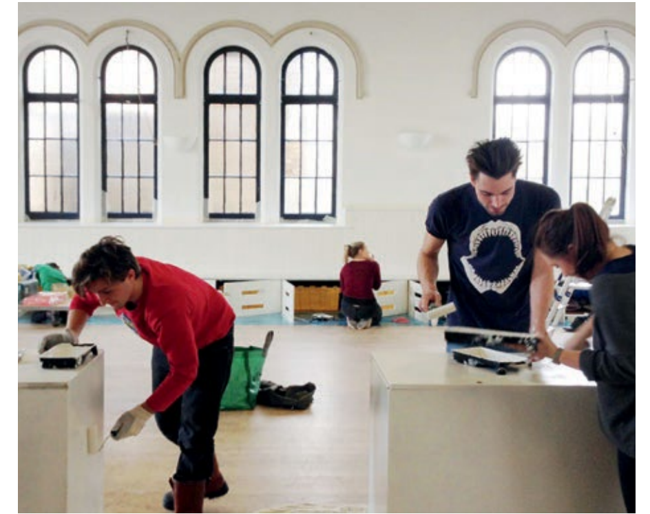
In October, a team of 15 took part in a hands-on volunteering day in support of community engagement charity Groundwork London. The volunteers worked on improving the indoor and outdoor environment of the Roundchapel community centre in Hackney.
